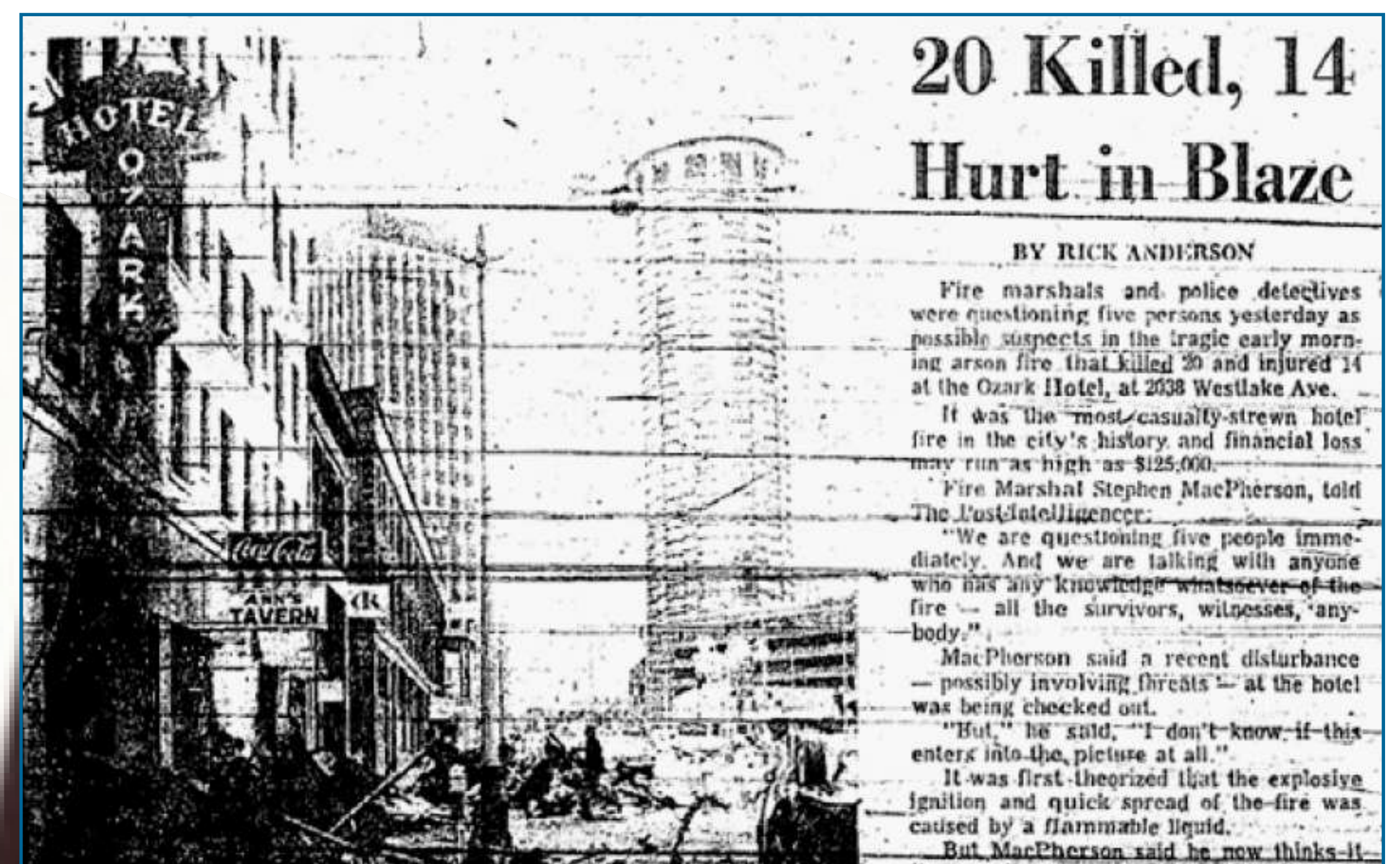
On the heels of two multi-fatality fires in downtown Seattle SROs, existing owners couldn't afford the required fire code upgrades, and vacated the buildings.
